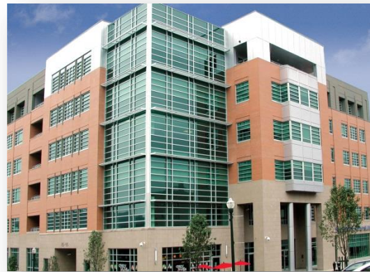
Figure 27: Southeast Curtain Wall
