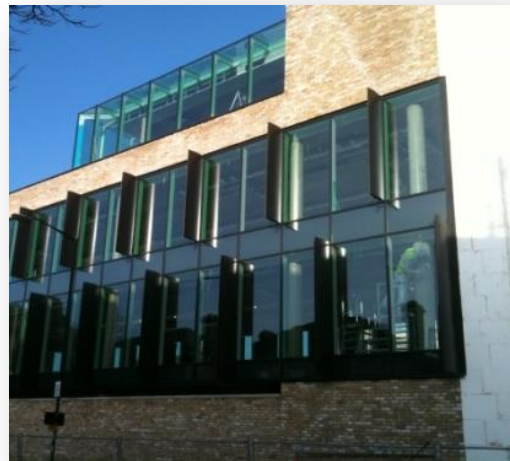
Figure 31: Vertical Shading Fins http://www.angarch.com/products/brise-soleil_01_archive.html
