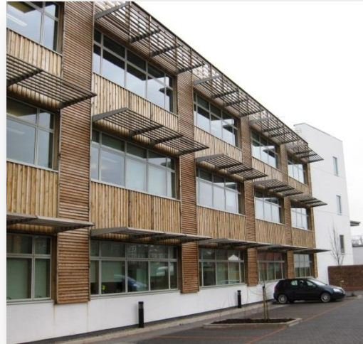
Figure 30: Horizontal Light Shelves http://levolux.blogspot.com/2012_02
